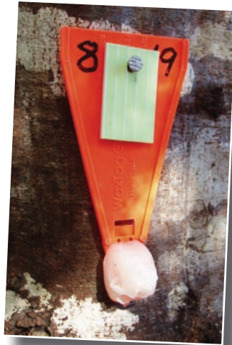
WaxTag® in position nailed 20cm above ground level.
